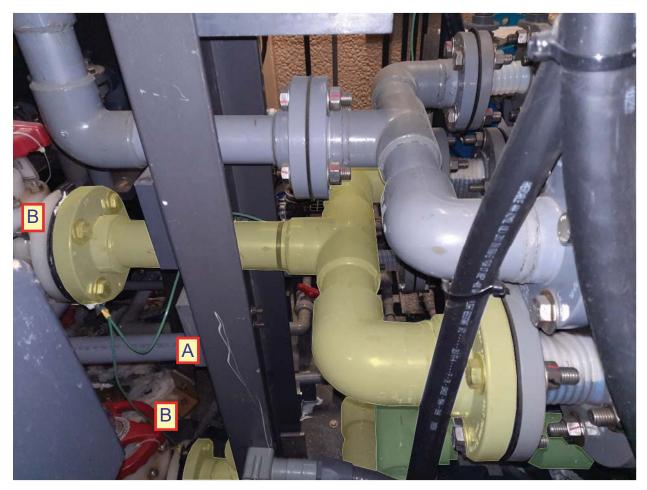
Grind out the support plates (A) as needed to prevent pipe from binding in the plate. Replace existing diaphragm valves (B) with new butterfly valves, stem mounted horizontally. Levers to be on side that will the operator the best access. New CPVC pipe is highlighted in yellow; new PP-RCT is highlighted in green.
