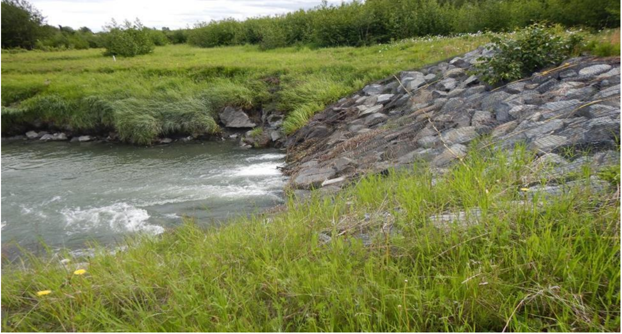
Figure 3: Culverts and rip-rap embankment for proposed removal.
