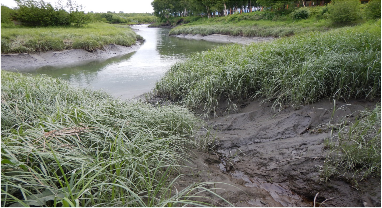
Figure 3: Bank stabilization area, looking towards Campbell Creek. The drainage in the foreground will be lined with a drain pipe and rip-rap apron.
