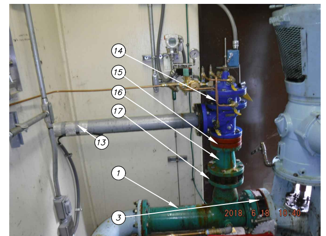
D EXISTING 3" PRV - ANGLE STYLE NOT TO SCALE
