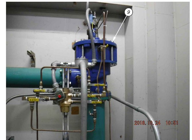
(G) EXISTING 6" BLOW-OFF PRV
