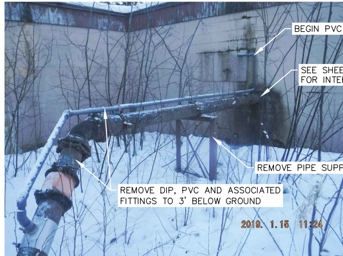
(B) EXISTING DISCHARGE CIP
