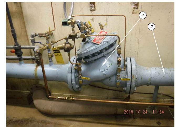
E EXISTING 8" PRV - GLOBE STYLE NOT TO SCALE
