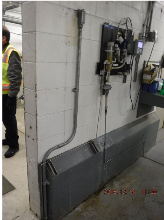
Photo 9-3: Existing Chemical Analyzer
