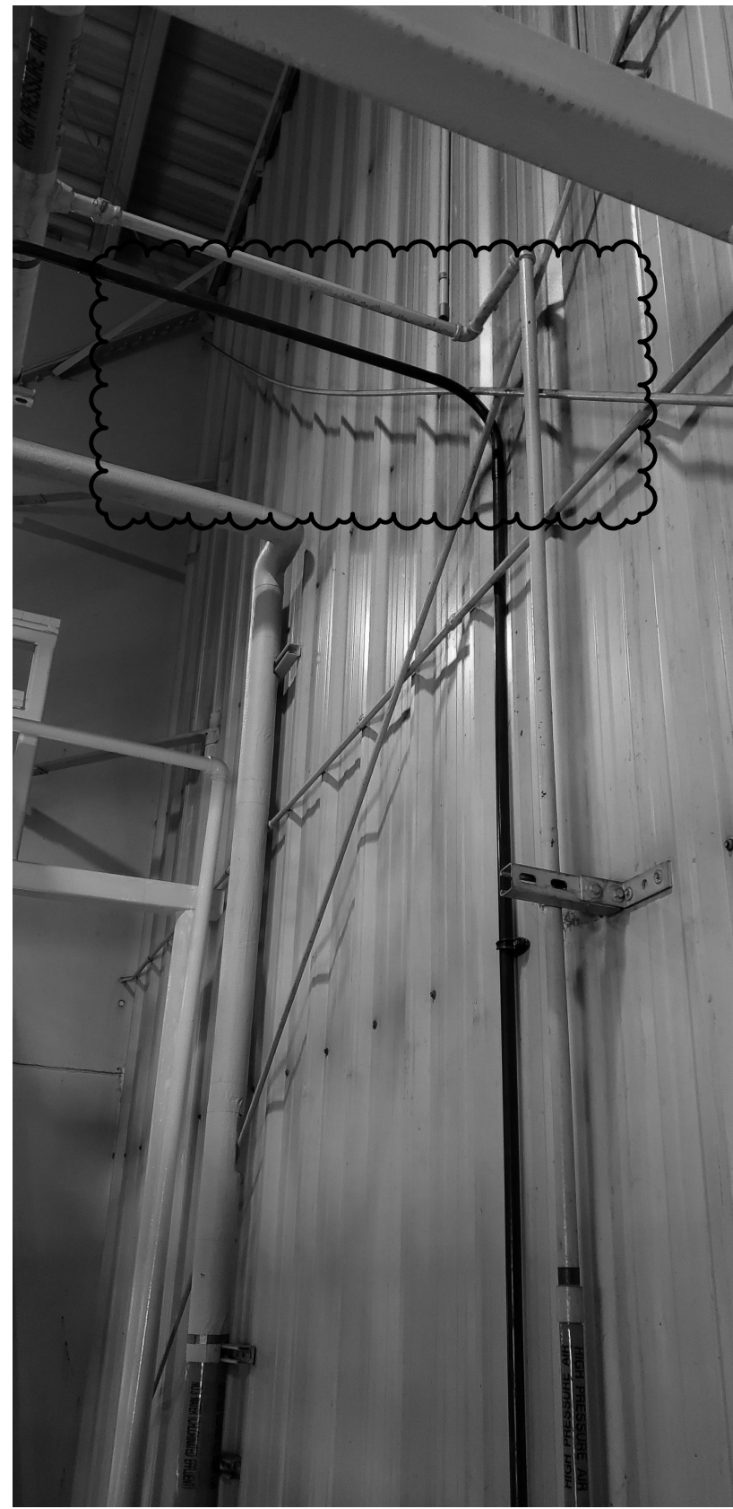
1 ELONGATED BRACES AT OCBF SCALE: NO SCALE
