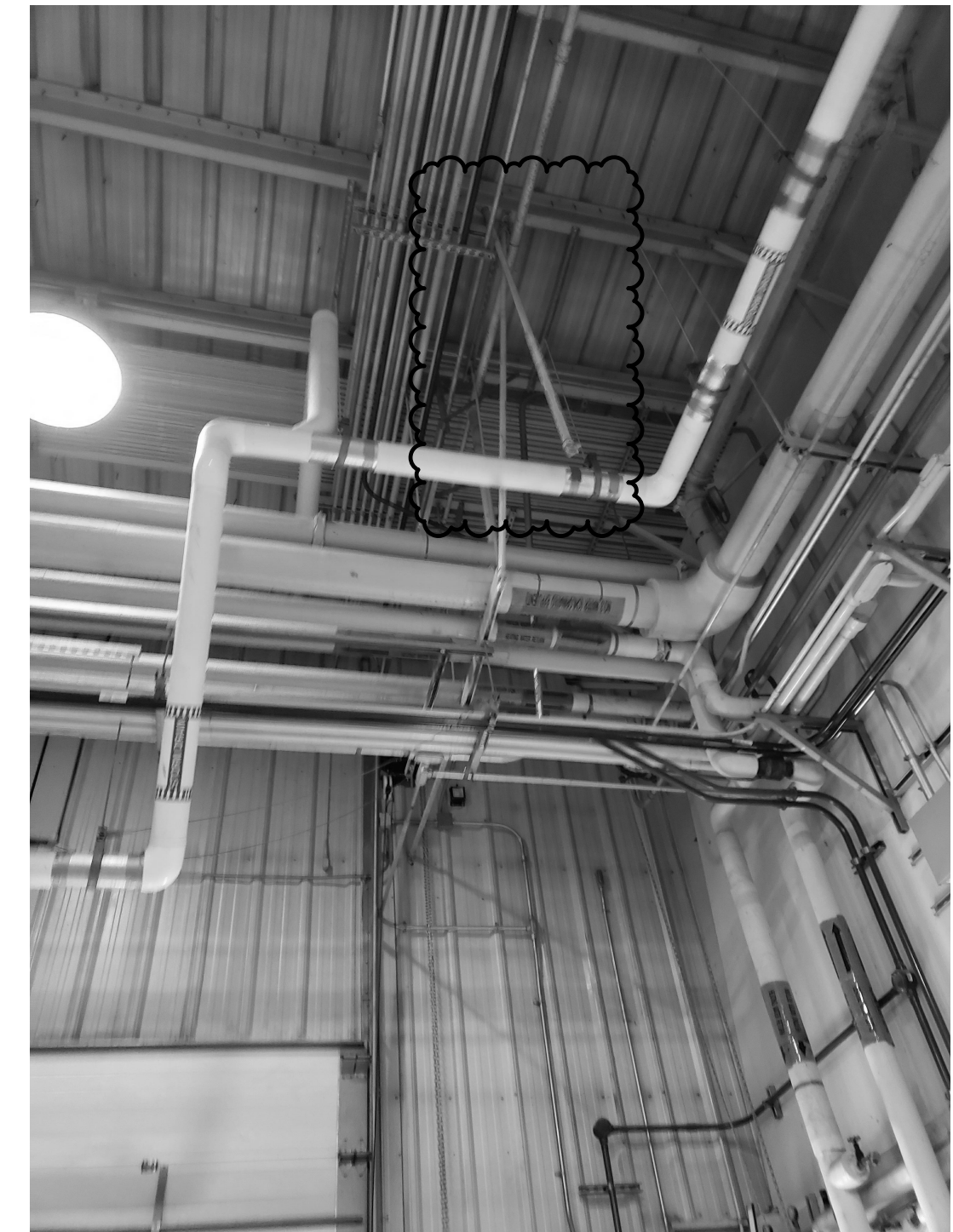
12 DAMAGED PIPE BRACING SCALE: NO SCALE
