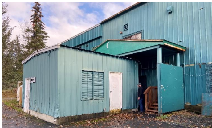
Photo 2 – Existing Generator Building – South Elevation
