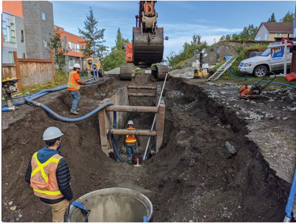
Photo 1: View looking north into excavation where contamination was first discovered. (August 27, 2020)
