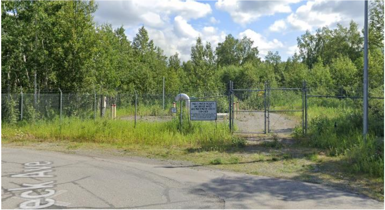
Robert Rude PRV Station - 9101 Peck Ave
