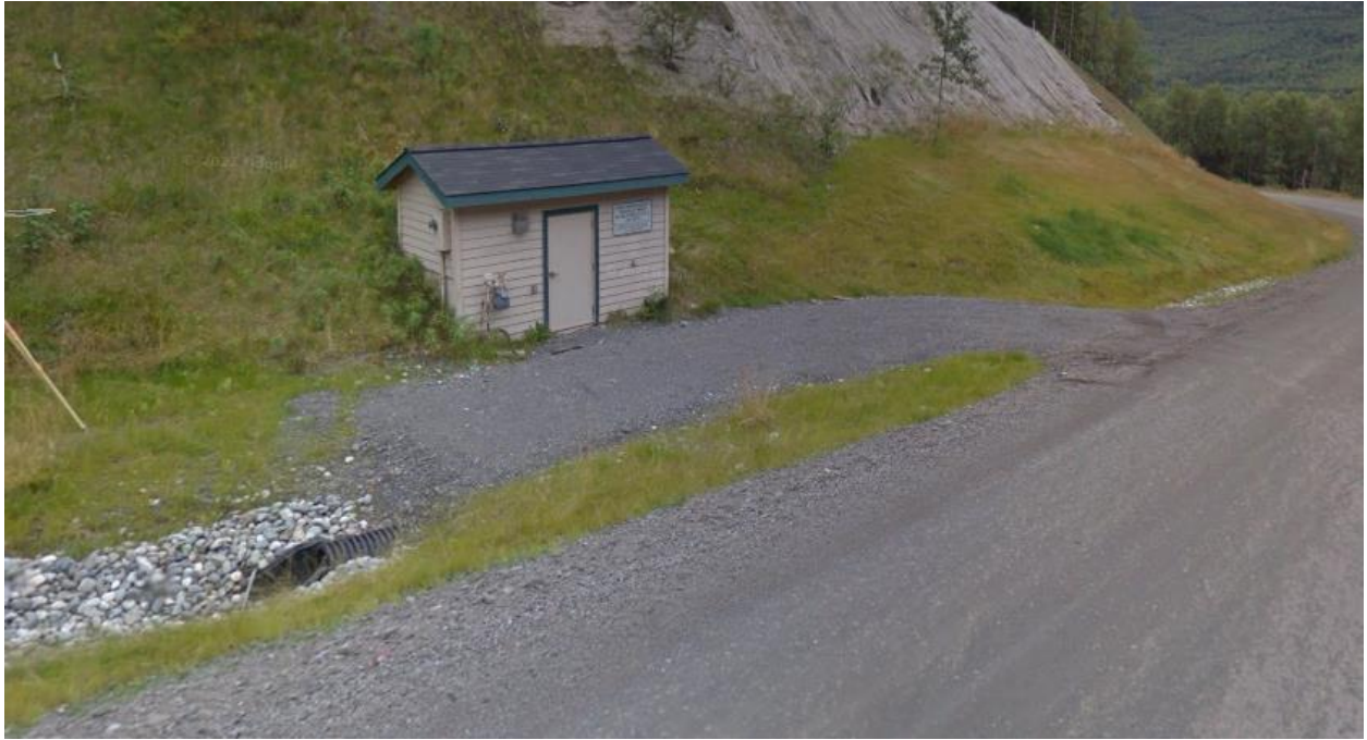
Eagle Crossing Upper PRV Station - 9425 Eagle River Ln
