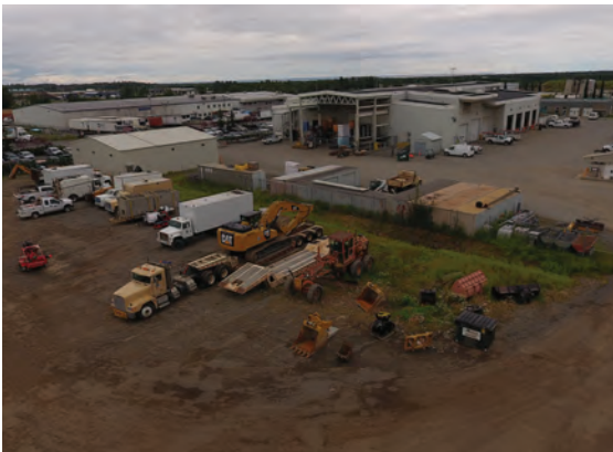
Figure 18: Overflow parking of fleet vehicles and storage connexes constrain the middle of the site
