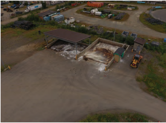
Figure 17: Grit Handling Facility
