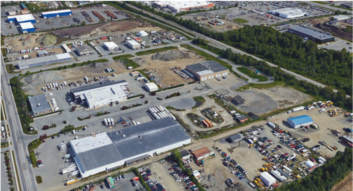
Figure 01: Aerial of King Street O&M Campus from Southwest
