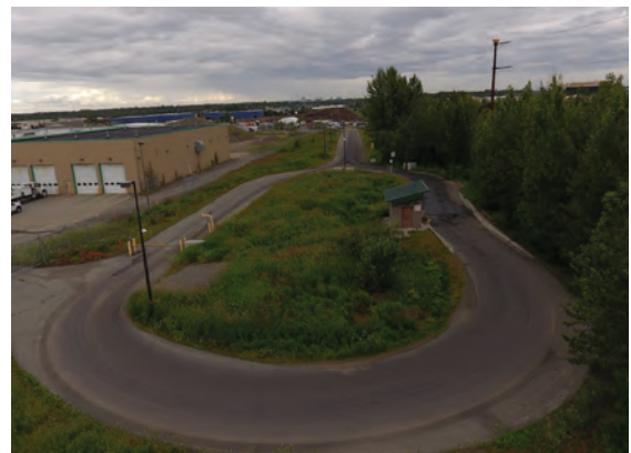
Figure 16: Septage Receiving Facility
