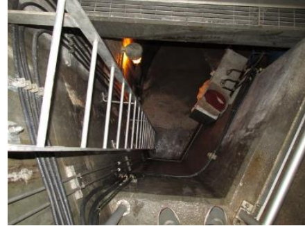
Figure 2-12 Sump Access Ladder
