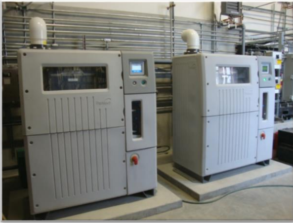
Figure 4-40 Miox existing installed 2X300 ppd Rio units [Parkson] (left), and Miox cassette-style vertical electrolyzers [Parkson] (right)
