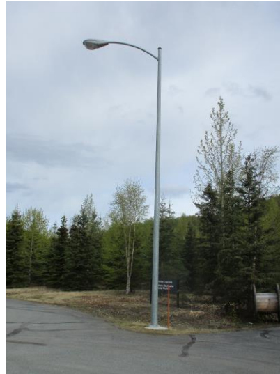
Figure 2-30 Pole Mtd Fixture
