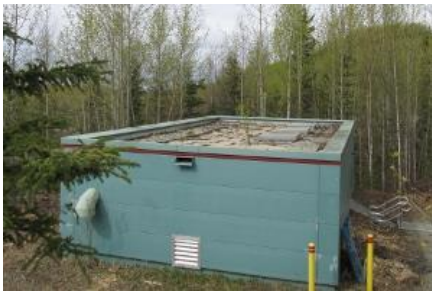
Figure 2-2 WWPS Existing Roof
