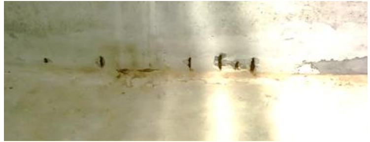
Figure 2-17 Exposed Rebar
