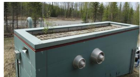
Figure 2-3 Effluent Vault Existing Roof
