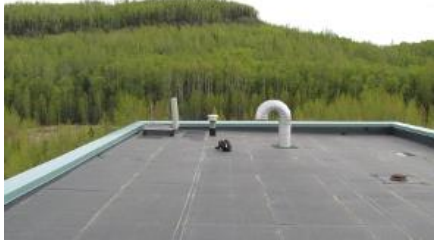
Figure 2-4 Primary Coagulant Tower Roof Access
