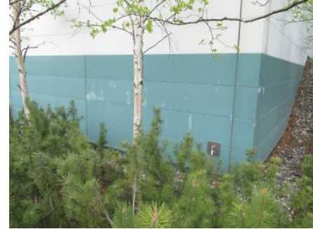
Figure 2-1 Typical Exterior Panel Discoloration
