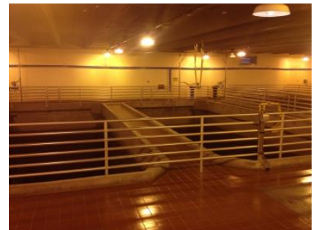
Figure 2-8 Typical Filter Basin Guardrail
