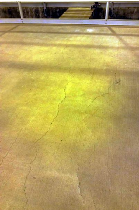
Figure 2-15a Floor Cracks
