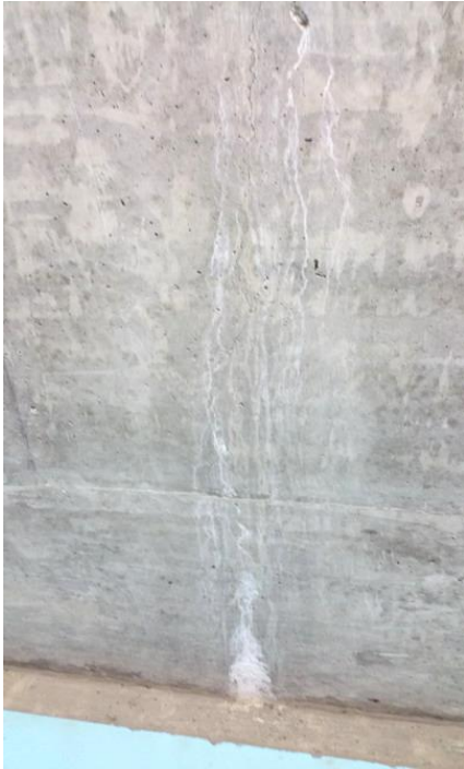
Figure 2-16 Wall Cracks
