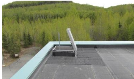
Figure 2-5 ERS Roof Access
