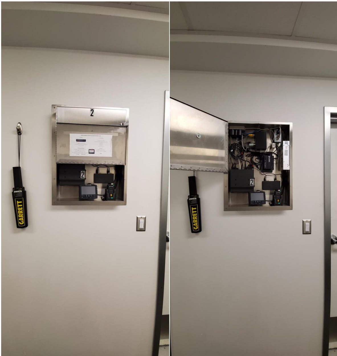
Control Panel outside of Interview Room, houses the DVR, WG Control Panel, Wireless Mic and all Electronic Wiring Components.
