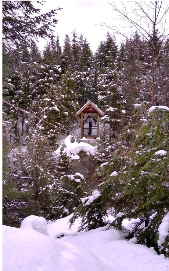
Existing Tram, Looking East (Feb 2021)
