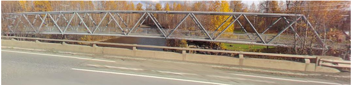
Figure 13 EXISTING PEDESTRIAN BRIDGE AT MONTANA CREEK
