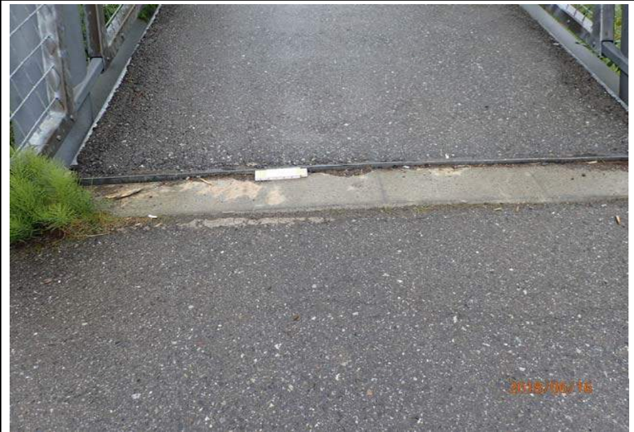
Bridge No. 6012 Br. Name Montana Cr Pedestrian Date 06/16/18 Inspector Sara Manning / Mary McRae Frame 12 Bump and spalls at NE joint File P6160145.JPG
