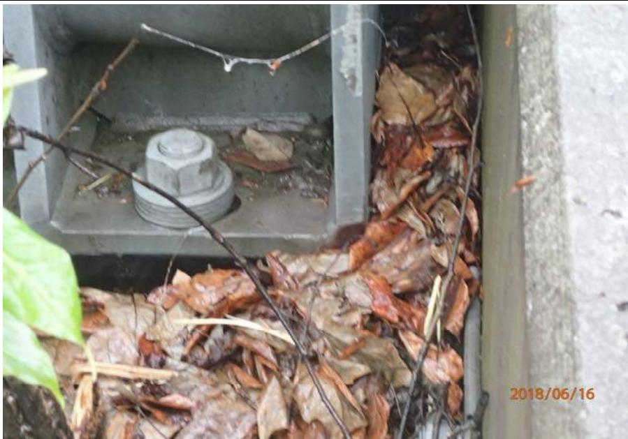
Bridge No. 6012 Br. Name Montana Cr Pedestrian Date 06/16/18 Inspector Sara Manning / Mary McRae Frame 11 Typical debris at exterior bearing (NE DS shown) File P6160134.JPG
